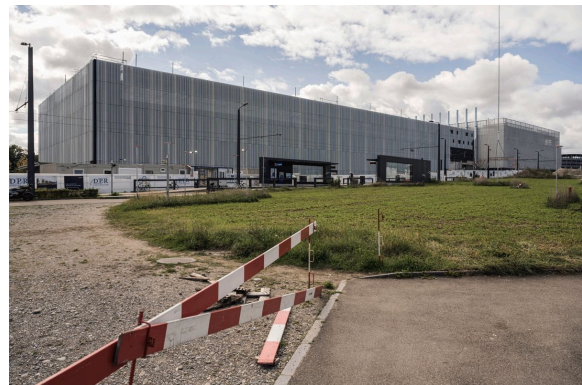
DATA CENTER ZUR 2&3, DIGITAL REALTY GLATTBRUGG. Photograph: AOT, 2025
