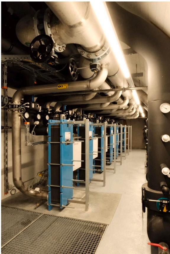
Water-to-water heat exchanger.
