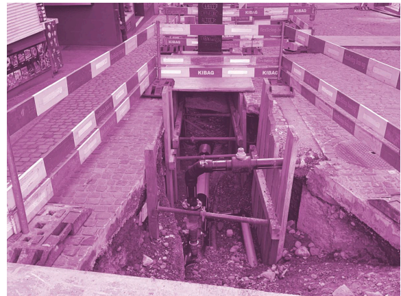
LAYING OF GAS PIPE
