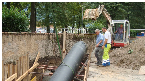
Laying of cooling pipes. Source: hpc-ch YouTube, 2011.
