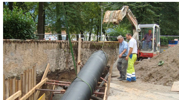
Laying of cooling pipes. Source: hpc-ch YouTube, 2011.
