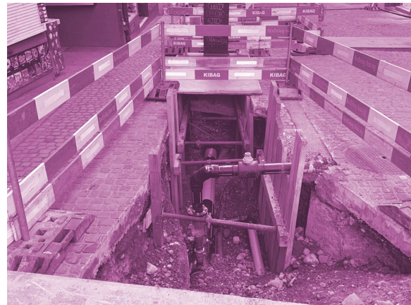
LAYING OF GAS PIPE
