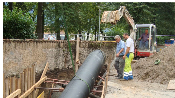
Laying of cooling pipes. Source: hpc-ch YouTube, 2011.
