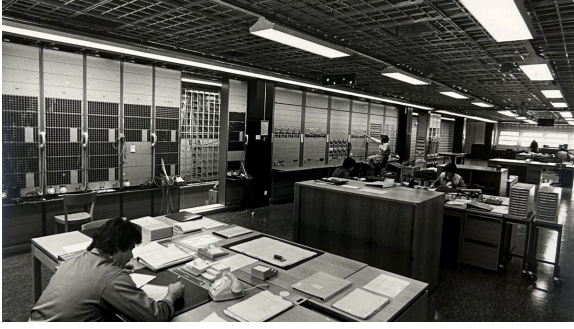
People working in the telecommunications centre of Herdern. Source: gta Archive, ETH Zurich.
