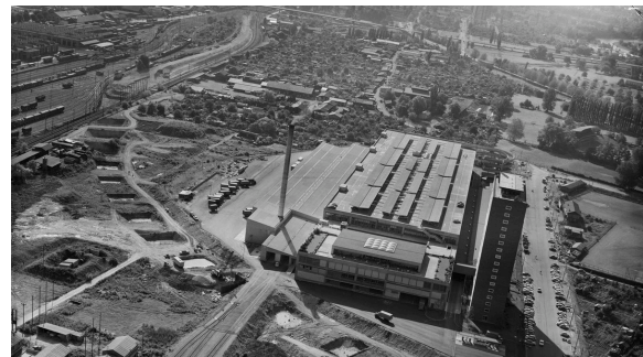
Aerial View of the Migros Building, 1965. Source: Sozialarchiv Zürich.
