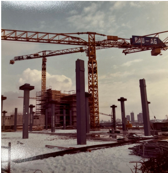
Construction site of the FBZ III, 1975. Source: gta Archive, ETH Zurich.
