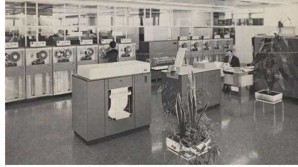
Inside the Postal, telephone and telegraphy services (PTT) Ostermundigen, parts of the IBM Computing System, 1968. Source: die Post.
