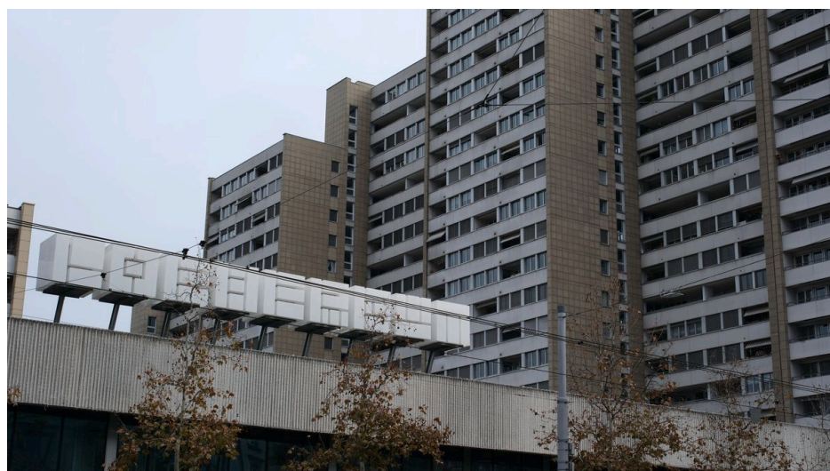
LOCHERGUT RESIDENTIAL COMPLEX. Photograph: film still from Wohnsiedlung Lochergut , video by the authors, 2025.
