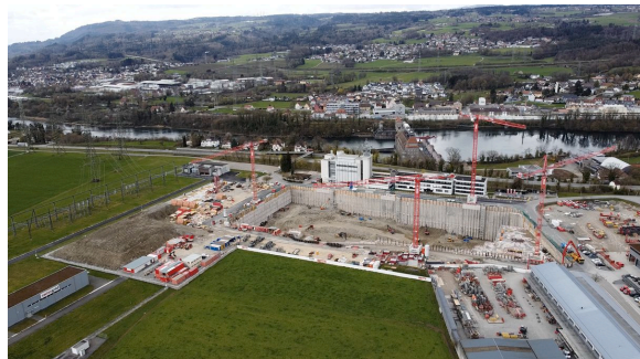
Construction of Flexbase, ongoing.
