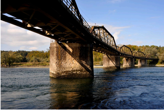
SBB Aarebrücke Koblenz connecting Basel to Romanshorn, built 1892. Source: Wikimedia Commons.
