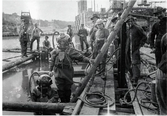
Construction of the hydro powerplant Laufenburg, 1909–14.
