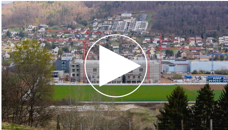
Data Centre Beringen: An Isolated Object in the Landscape , video essay, 2026. https://www.youtube.com/watch?v=-9YrsU5KSaE
